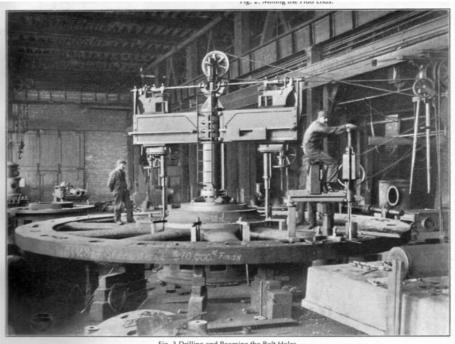
Fig. 3 Drilling and Reaming the Bolt Holes.
